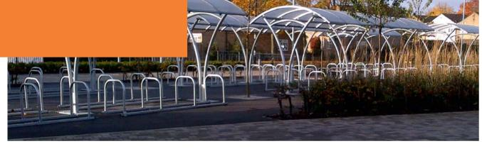
Cycle shelters are essential to modern transport infrastructure, providing protection from the elements for cyclists at work, in education and on the move. Typically situated within a secure site, cycle shelters are open type structures, clad in clear polycarbonate for glass to limit visual impact and maintain clear lines of sight through the cycle parking facility. Cycle shelter cladding options include timber slat, glass and decorative laser cut steel vision panels.
